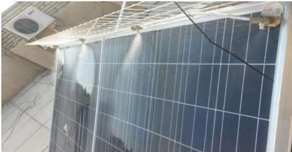
Figure.6 PV panel and network of mist nozzles
